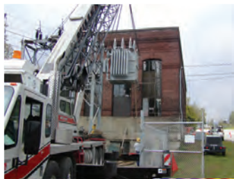
Rigging a new GSU transformer
